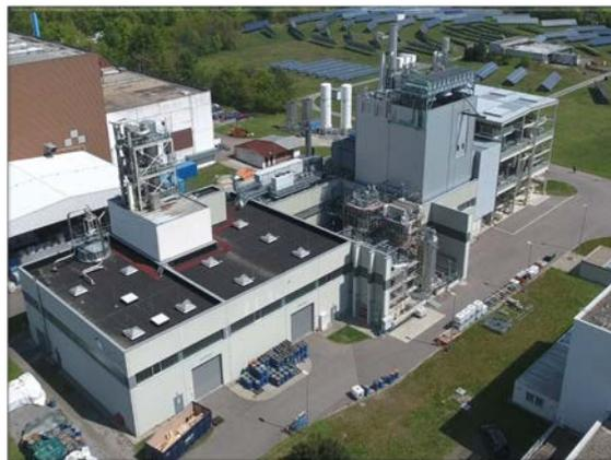
Afterwards, the workshop participants visited the *bioliq® pilot plant at KIT*, a fully operational biomass to liquids project and research platform that demonstrates production of synthetic transportation fuel from low quality non-food biomass feedstock in the ton-scale.
